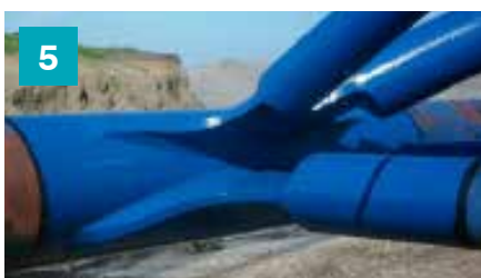
Complete post weld actions, apply corrosion protection coatings
