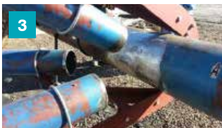
Prepare lacing ends and main chord surface for welding
