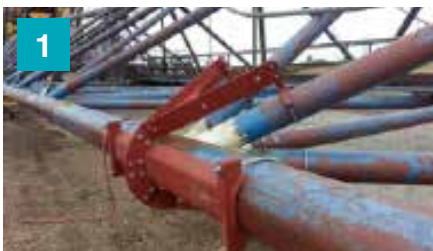
Attach engineered bracing to maintain geometry
