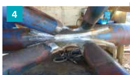
Weld new members
